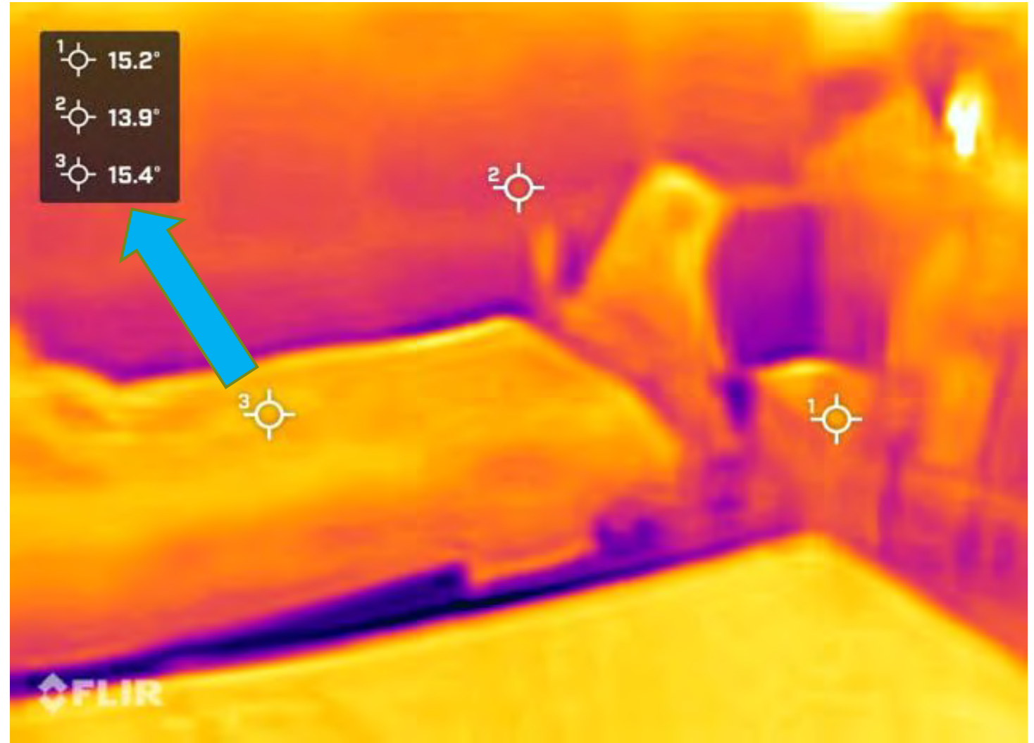
Pic Above: Shows a temp of 15.4 degrees – by repositioning bedding.
